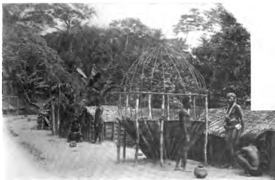
CONSTRUCTION OF A NATIVE STOREHOUSE, TURUMBU.
