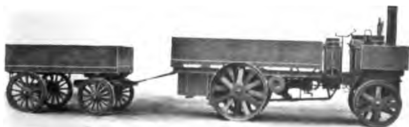
STEAM MOTOR WITH TRUCK.
