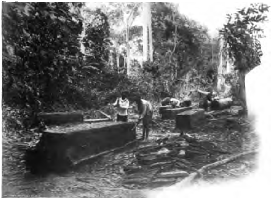
SHAPING TIMBER BY HAND.
