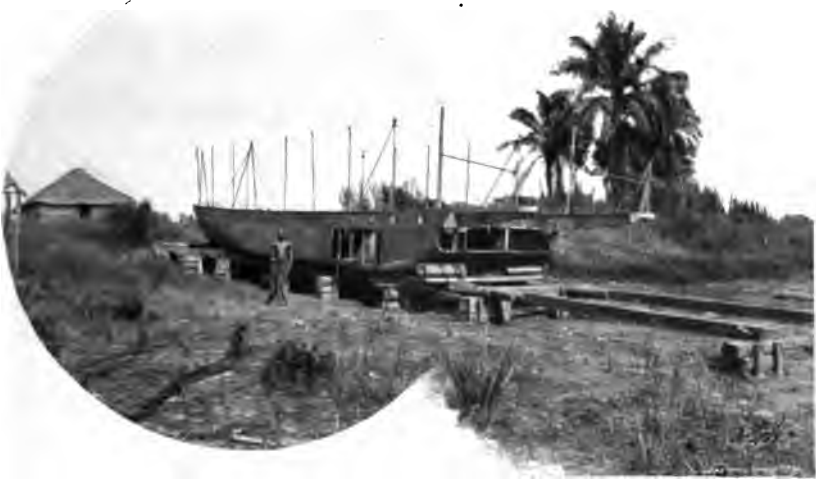
SHIPBUILDING AT LEOPOLDVILLE.
